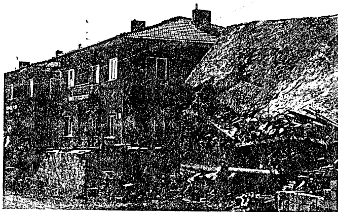
FIG. 42. Example of older residential URM masonry buildings which have survived intact, next to a new building collapsed while under construction.
