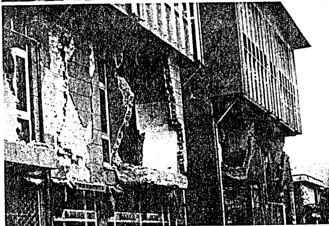
FIG. 28. Crushing of hollow brick masonry and separation of infills from the frames.
