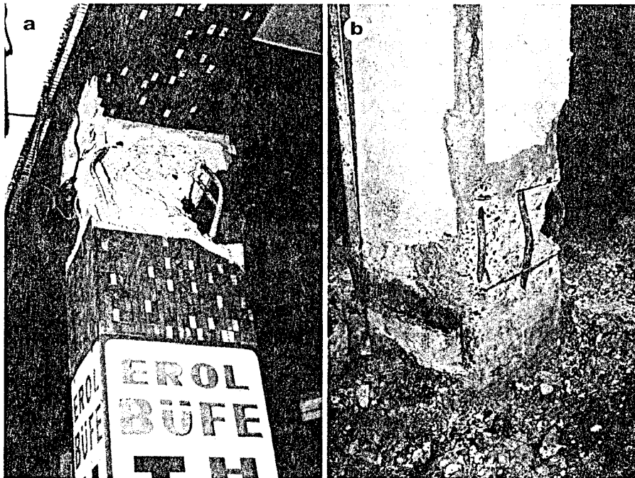
FIG. 14. (a) Lack of column confinement and buckling of longitudinal reinforcement in the first storey of a commercial building in centre town; (b) lack of column confinement in Sumerbank Textile Factory.
