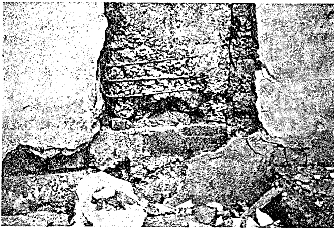
FIG. 24. Lack of reinforcement detailing in a beam-column joint with beam offset.
